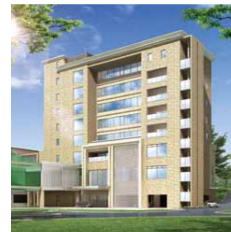
Hotel Tado Onsen Residence New Annex
